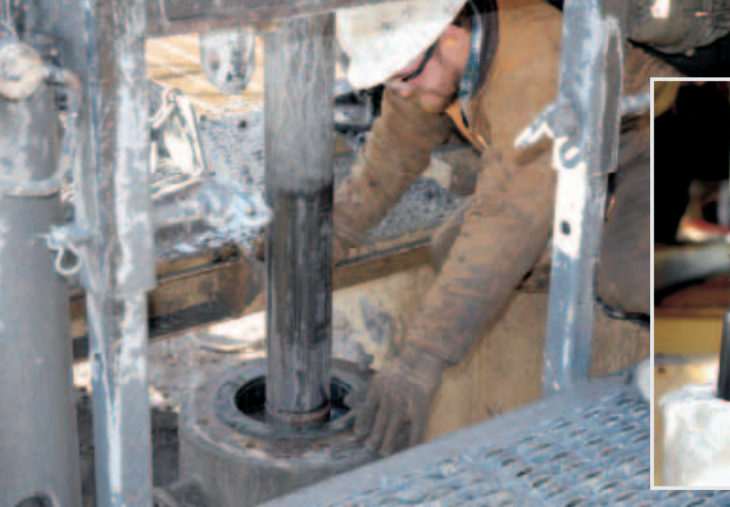
After the hammer and stabilizers have drilled deep enough into the hole to clear the surface casing, the collar is set in place, forcing the cuttings, water and gas through the discharge line.
